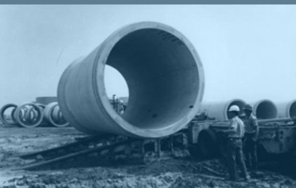
1947 Construction of a 7,000 foot long ocean outfall using 78-inch diameter pipes.
