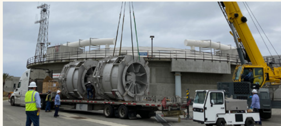
Major equipment replacement at Plant No. 2 to maintain reliability.
