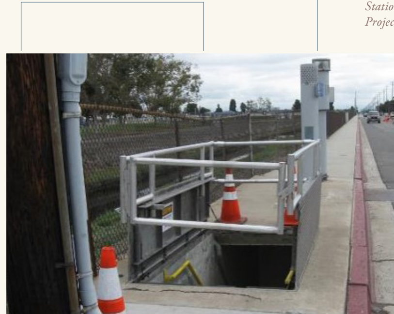
The existing Edinger Pump Station is located completely underground and accessed through a hatch that requires the closure of the sidewalk along a school and park.
